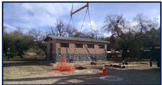
Prefab restroom being installed in the Hassayampa River Preserve
